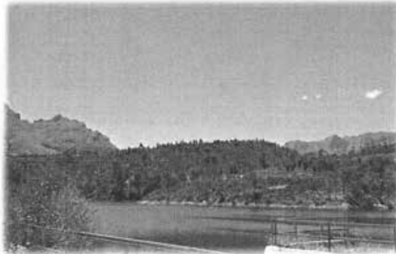
Figure 5: Idas Valley Dam 2.
