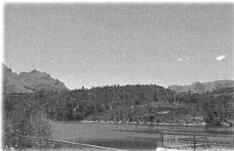
Figure 5: Idas Valley Dam 2.
